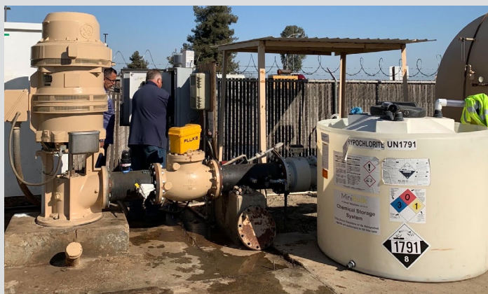
Picture: Tulare tests new pump efficiency after installation on Well 25
